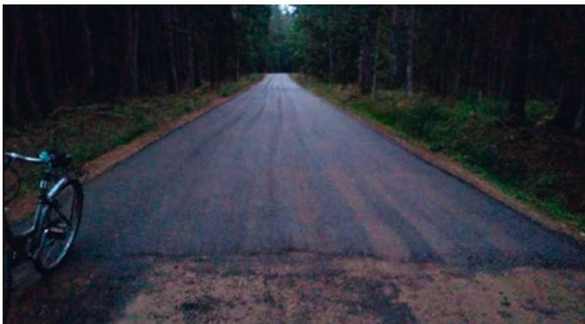
*Fig. 26: Previously forest ground road being upgraded with a bituminous layer*
